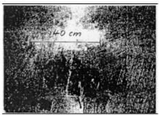
Fig. 37: Inky blue stains on the plaster of a church fumigated with hydrogen cyanide.
