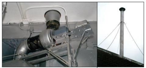
Fig. 102: Exhaust fan and stack on top of gas chamber. Fig. 103: Exhaust stack.
