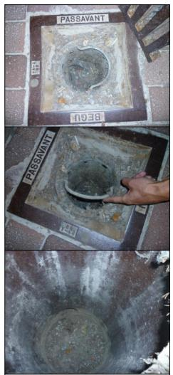
Fig. 61a & b: One of the six floor drains inside the alleged gas chamber at Dachau. Left: grate removed, sieve in place; right: sieve removed; the exit drain pipe can be seen at the drain's bottom (topmost spot of the bottom).
