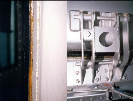
Fig. 104: Closeup of rubber seal around gas chamber door, also covered in Vaseline when in use.
