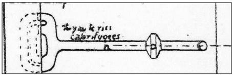
Fig. 56: Alleged design of the pipe in the attic area above the gas chamber. Air enters through a chimney extending over the roof on the right, then runs through a heat exchanger connected to the building's steam central heating. Shortly before the wall the pipe splits into two, then into four pipelines, only to merge with itself on the other side of the wall. (Part of a sketch by Captain Fribourg, Dachau archival no. 3407)
