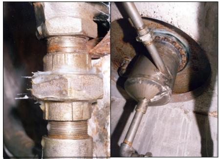
Fig. 106: Closeup of plumbing underneath the gas chamber covered in Vaseline to indicate leaks.
