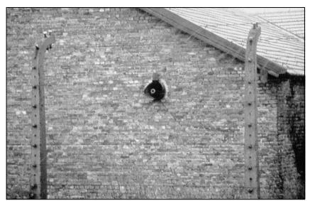
**Fig. 25:** One of the two ventilation outlets from the disinfestation wing of Building BW 5b, without equipment today. The other is located on the same wall slightly to the left. The end of a water pipe installed after the war is protruding out of the hole.
